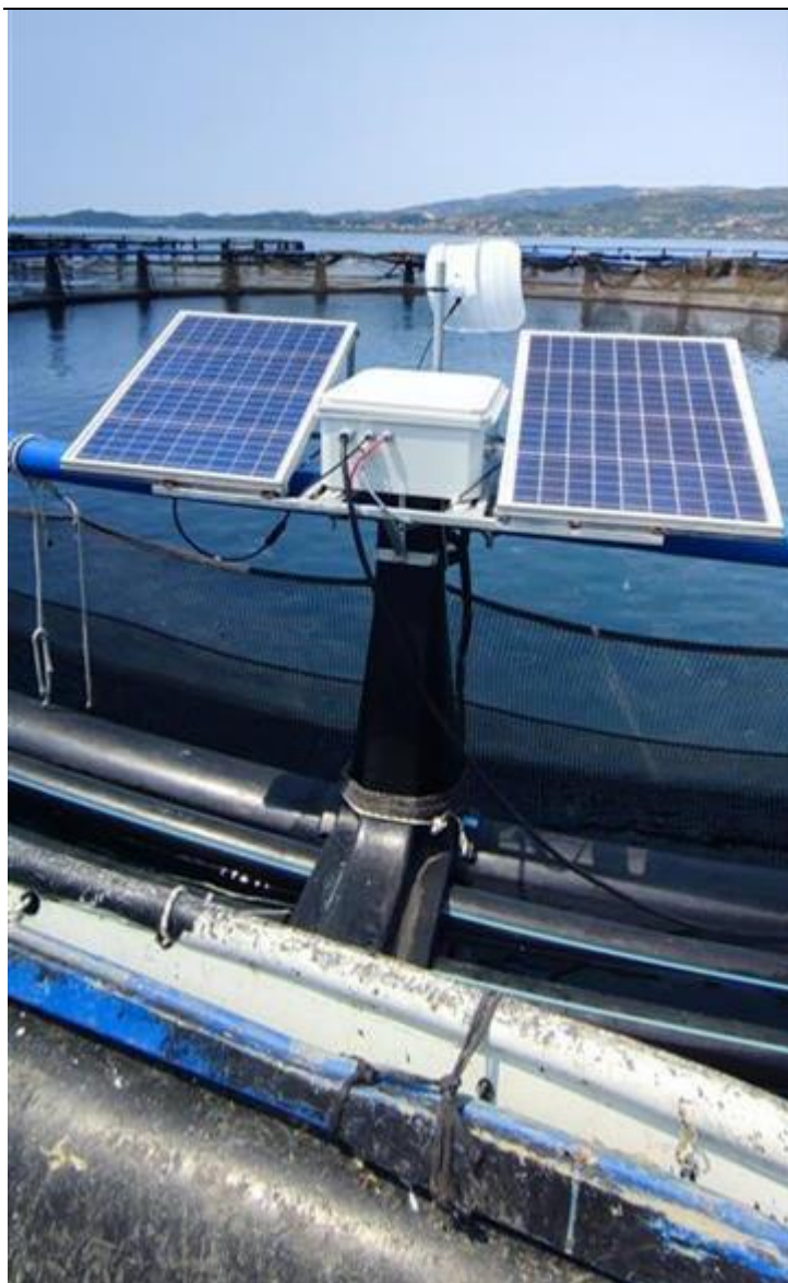
Figure 17: Solar panels were installed, attached to the mooring system
