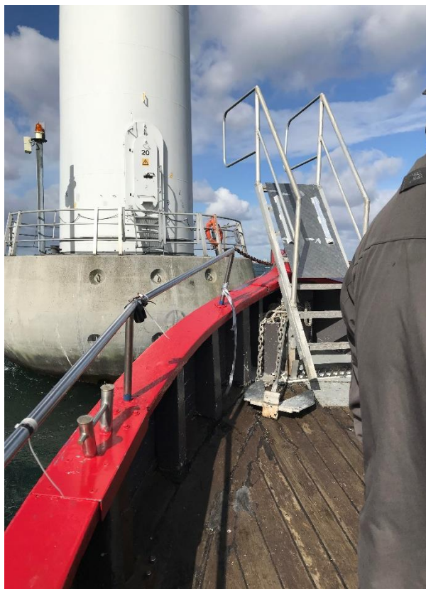
Figure 8 – Example of stairs used for direct access to the foundation
