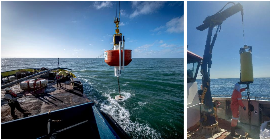
Figure 5: Difference between installation of the large data buoy with large vessel (left) and small data buoy with smaller vessel (right) at the Dutch pilot.
