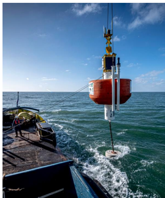
Figure 5: Installation big data buoy at the Offshore Test Site
