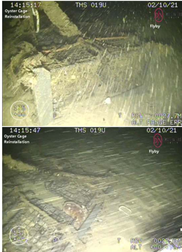
Figure 11 Survey image oyster structure 1 just before reinstallation with ROV 1- top: part which is not covered in sand, bottom: part which is covered in sand)
