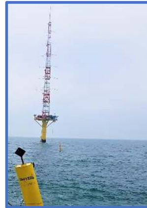
Figure 1 FINO3 research platform with aquaculture area in the front, located in the North Sea, Germany
